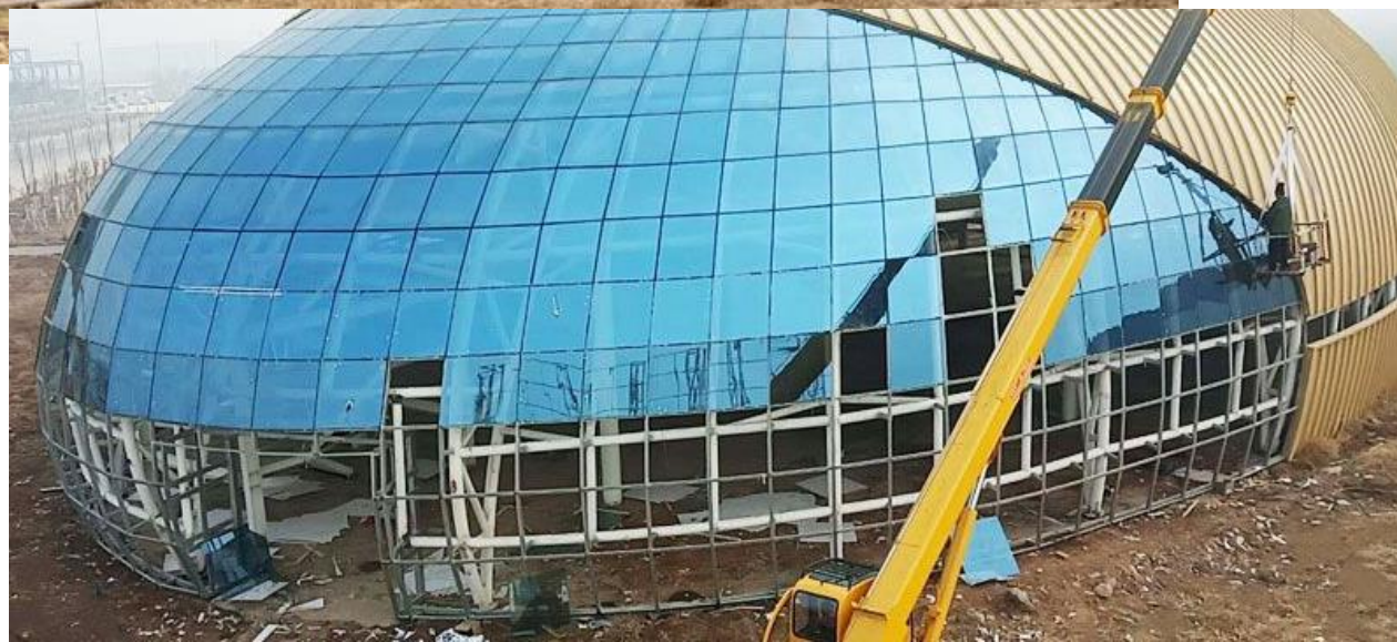
Girder dome (one-way), truss arches
