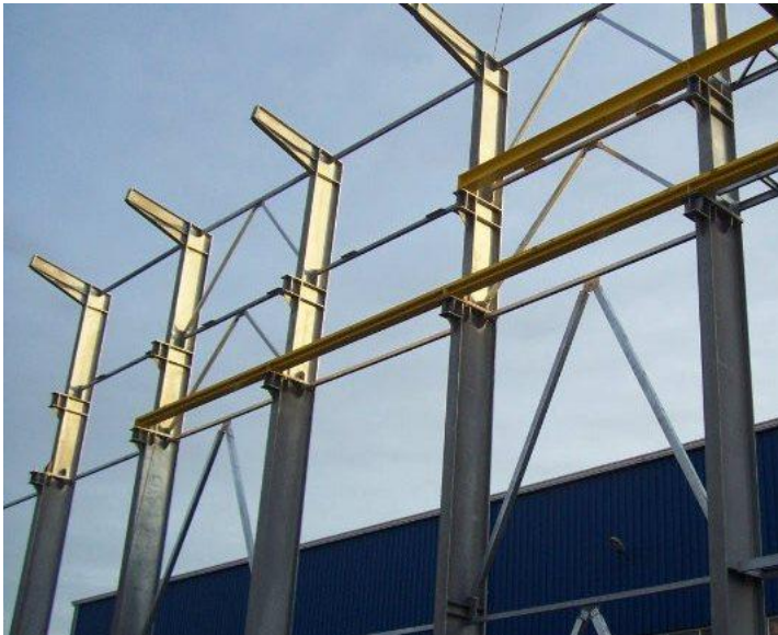
Cantilever, change of cross-section.
