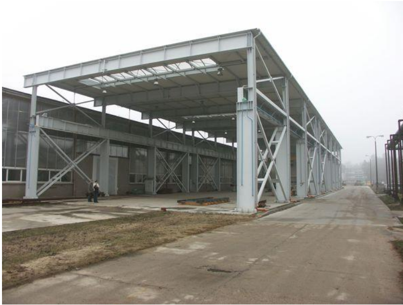
Welded I-column, change of cross-section.
