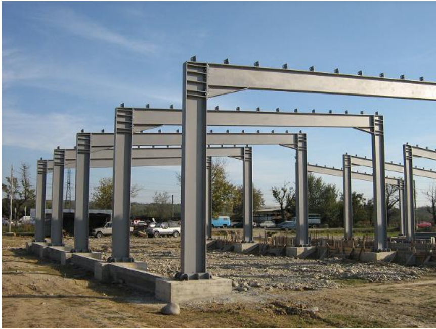
Photo: Setro Metal Group
