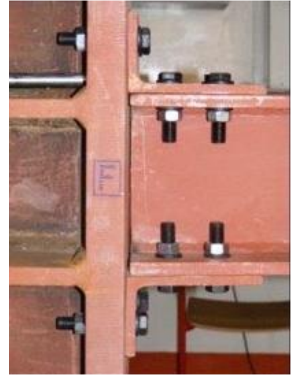
Photo: Behaviour of stiffened flange cleat joints, D. Skejic, D. Dujmovic, D. Beg
