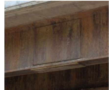
Welds between gusset plate and bracing or between flange plate and flange
