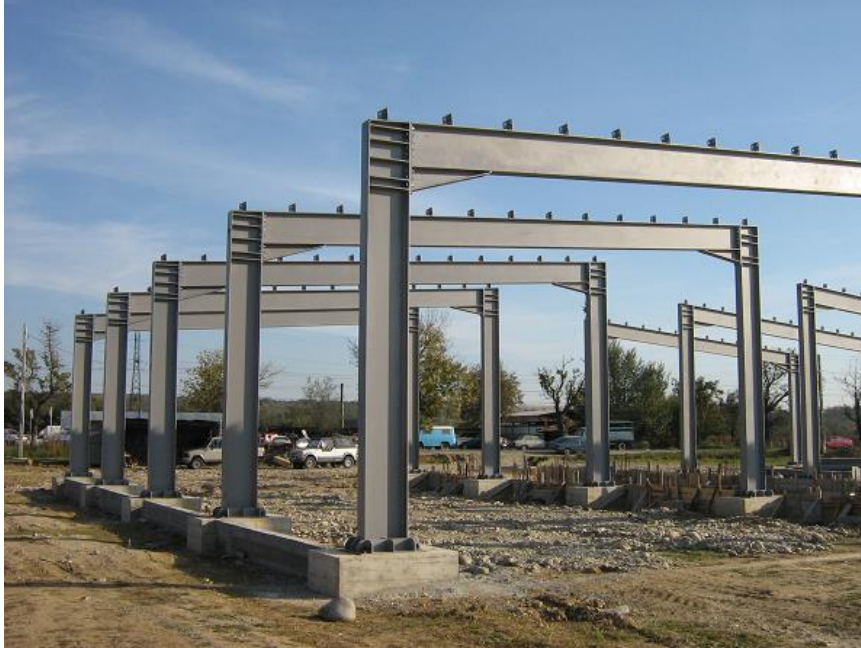
Photo: Setro Metal Group
