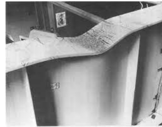
Photo: Web Buckling of High Strength Steel Plate Girders Induced by Bending Curvature, S. Nascimento, J. Pedro, A. Biscaya, Wiley Online Library, 9 III 2020
