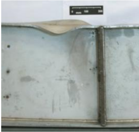
Photo: Saliba, N. Gardner, L. Experimental study of the shear response of lean duplex stainless steel plate girders. Engineering Structures. 1 / 2013
